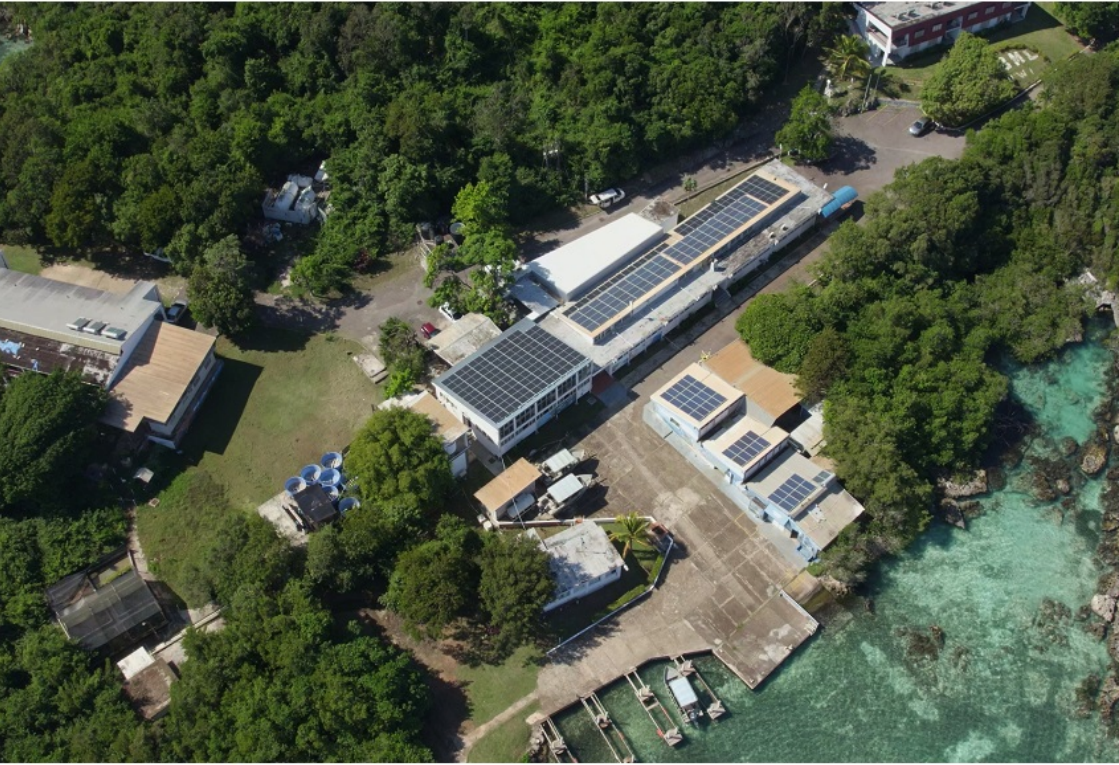
The 40 kW solar PV grid system installed at the Microgrid Training Centre.
